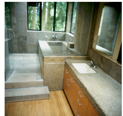
Antique stair treads and road pavers used as countertops and to build a Japanese style soaking tub.
