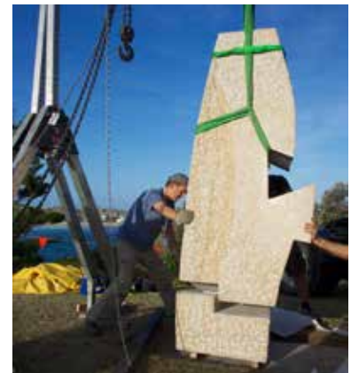
Installation images on site
