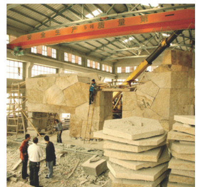
Sculpture pre-assembly for the Big Horn residence
