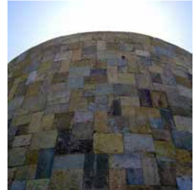
Antique Yangtze Limestone installed at the Keller Winery, CA
